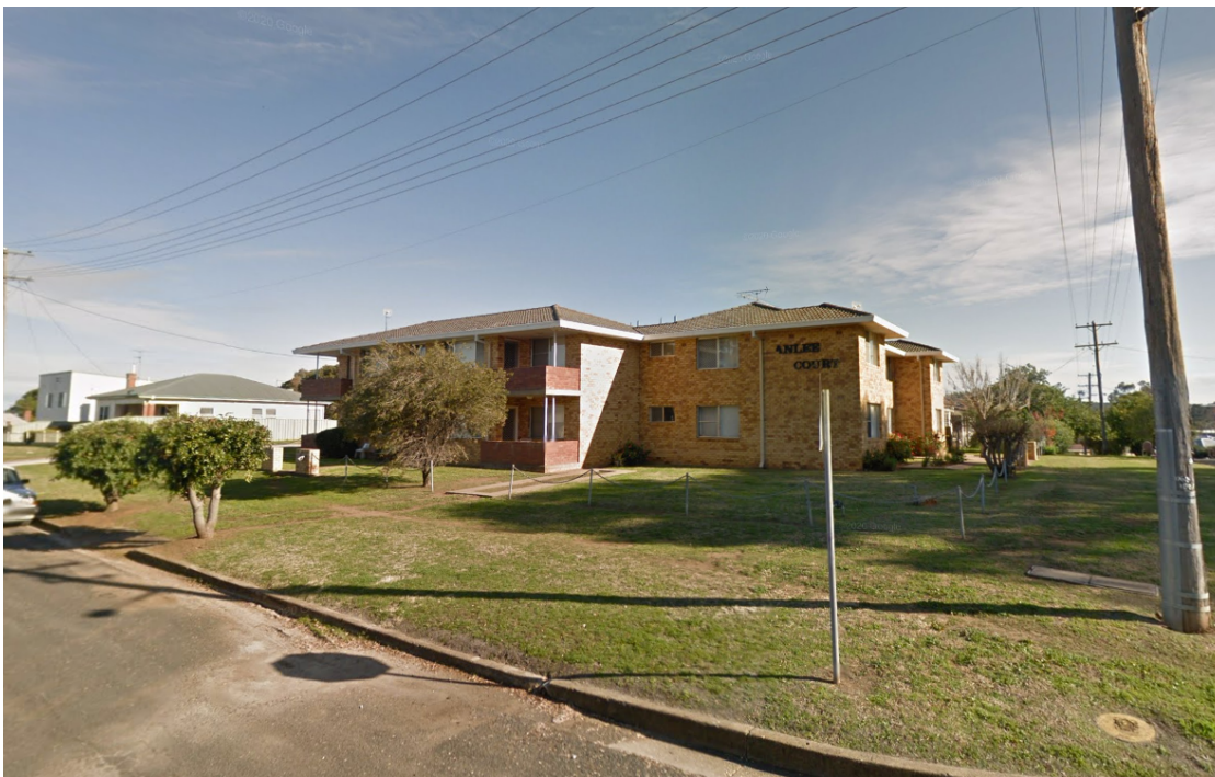
Photograph 3: Shows an older style two storey walk-up RFB located on the south western side of Upper Street (12-14 Macquarie Street, North Tamworth).
